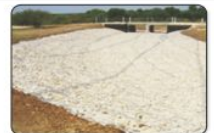
Bridge & Culvert Protection
